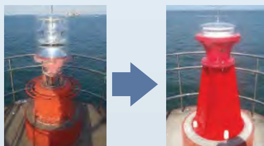
Reinforcing a light source against wave damage
